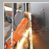
Quick saw & Chain Saw Breaching
